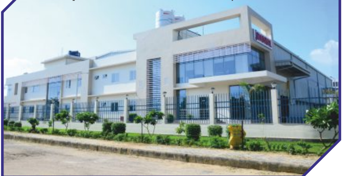
Bilaspur Works : Manifolds & Cylinders
