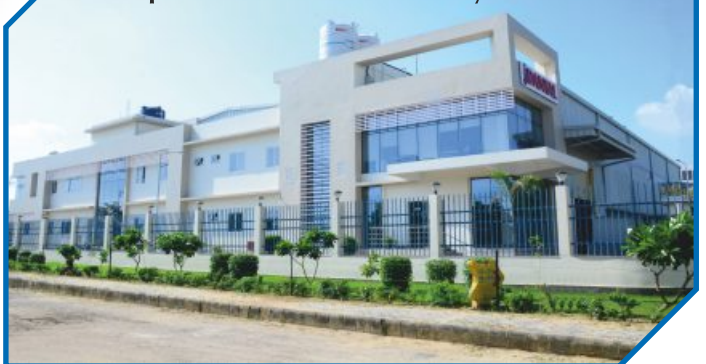
Bilaspur Works : Manifolds & Cylinders
