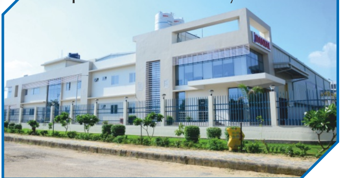
Bilaspur Works : Manifolds & Cylinders
